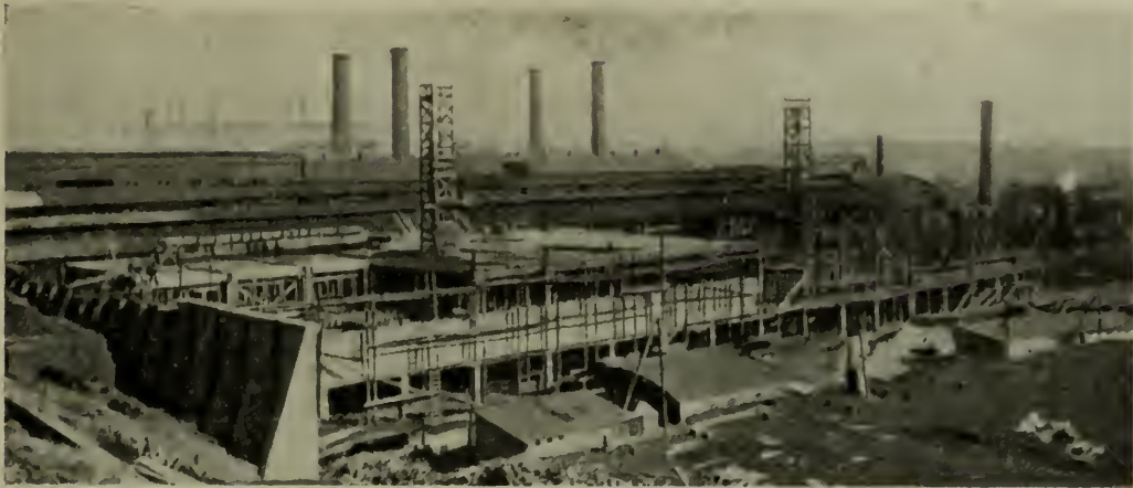
PROVAN GASWORKS : Works under Construction : Retaining Wall No. 2 on Left.
